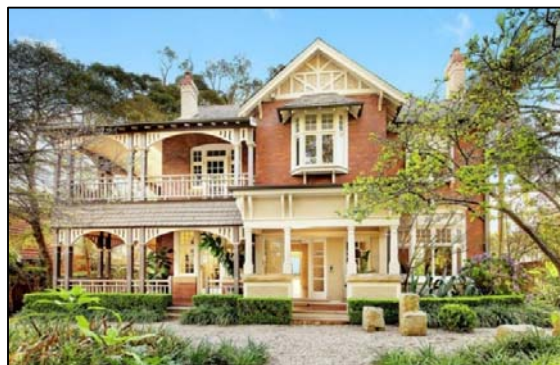
“Leesthorpe”, 20 Bradleys Head Road, Mosman
