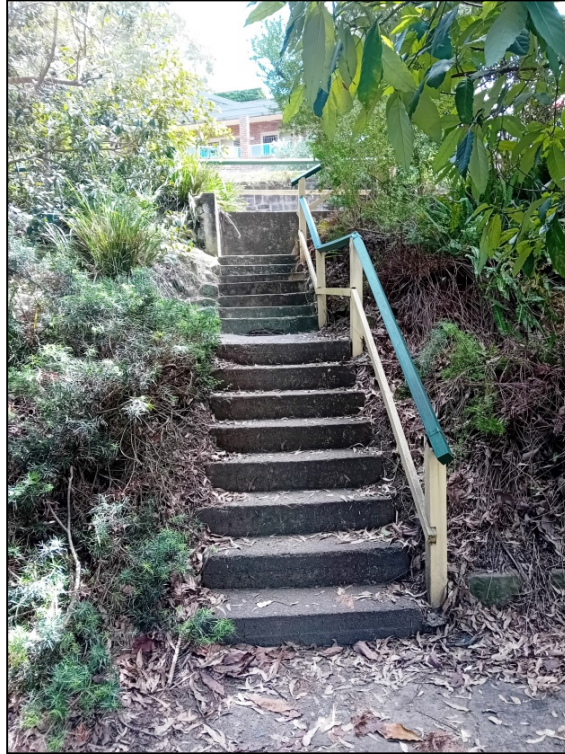
Steps leading down from Park Avenue towards Reid Park. (P Lofthouse, 2024)
