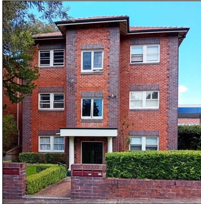
“Brierwood Flats”, 26 Brierley Street. (P Lofthouse, 2024)
