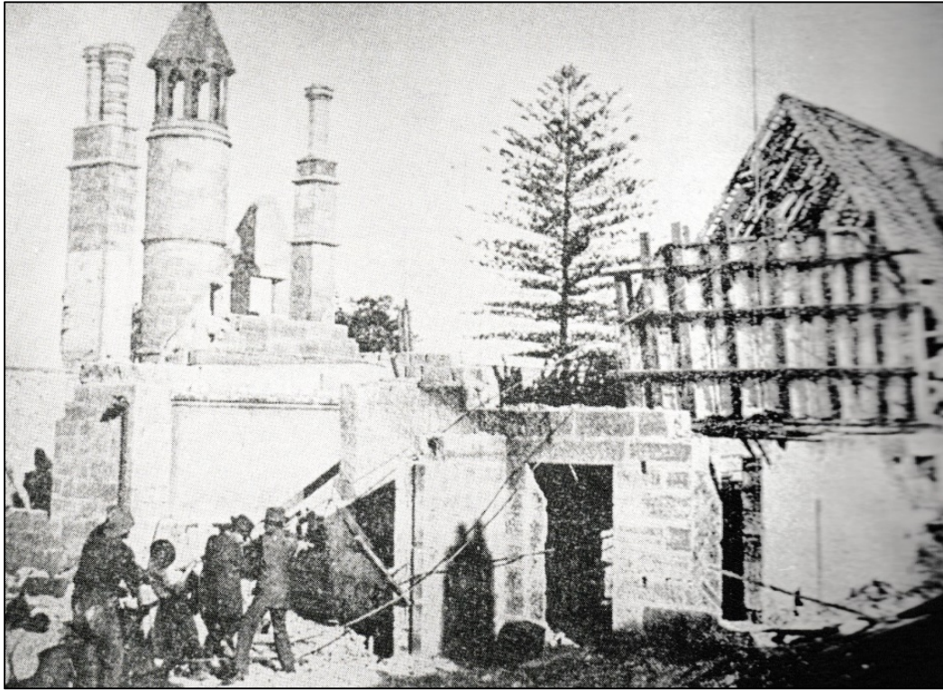
The wall with the drawing being removed. (Hughes, p118)
