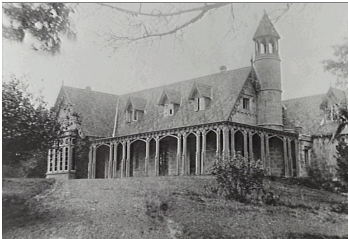
"The Rangers", 1914, just prior to its demolition. (Mosman Local Studies Library, Mosman Library Service)
