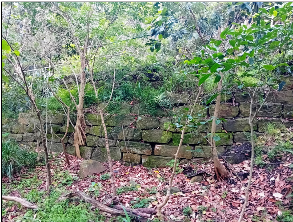
The lower wall is part of Bloxsome's original track. The current walkway above it follows the same route. (P Lofthouse, 2024)
