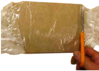
Plastic wrap on the Attic Partition - avoid bunches and wrinkles
