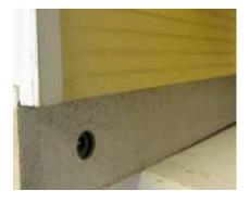
23. If your wiring is already in the cellar, good! Otherwise, Cut a slot for the tapewire using an oscillating Multitool or drill holes thru the floor to access the house wiring with the connection wire.
