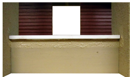
Foundation behind the Front Steps
