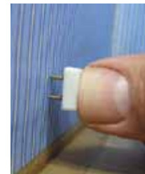
Mark it with the prongs of a plug
