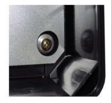
\*If you are in a very damp environment and concerned about water ingress, use some silicone on/around the lag screw during installation for extra sealing insurance.
