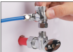
Connect the adapter and make sure the rubber O ring is loaded
