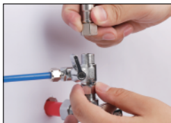
Connect the flexible hose
