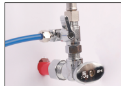
Valve installa on complete
