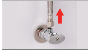
Remove the existing water hose
