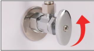
Shut off the water supply
