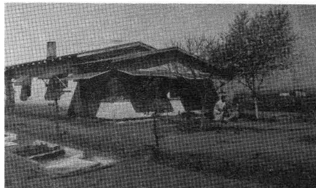
The historic Sylvester House property, pictured here in the 1920s or 30s, is the new NS/S office and garden annex.
