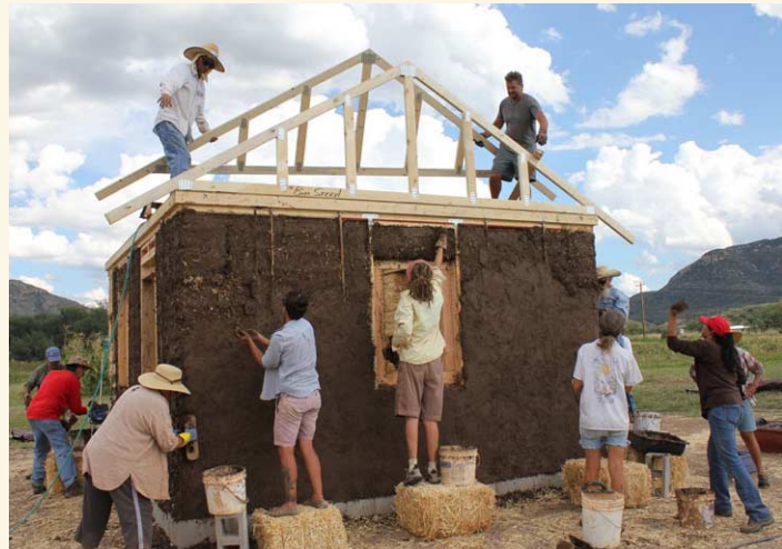
Below: Participants apply mud plaster and install roofing during a Straw Bale House workshop on the NS/S farm.
