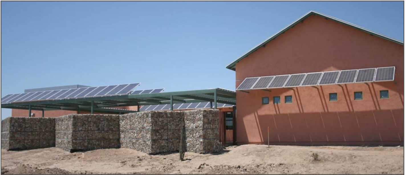
The southern elevation of our new Agricultural Conservation Center features photovoltaic solar panels donated by Tucson Electric Power and installed by Technicians for Sustainability. A courtyard is enclosed by the building's walls and a beautiful gabion wall.
