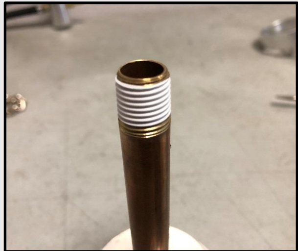
Wrap threads with PTFE thread sealing tape. 2-3 wraps will be sufficient
