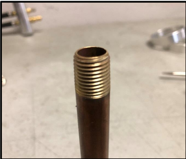
Make sure threads are clean of debris and old sealant
