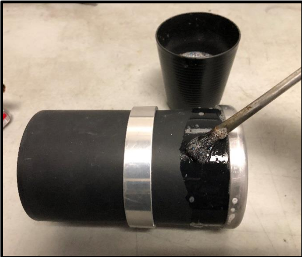
Lubricate the bladder heavily with soapy water
