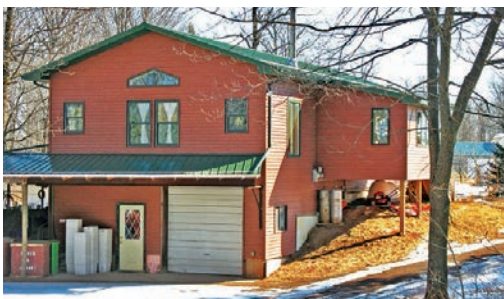
Figure 6. Modern root cellar in the lower level, below office or living space. Food Farm in Wrenshall, MN. (Courtesy of Janaki Fisher-Merritt)
