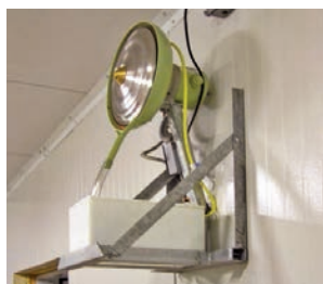
Figure 31. Commercial-capacity centrifugal humidifier. (Sanford)
