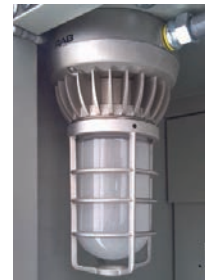
Figure 18. LED wet-rated jelly jar style ceiling fixture. (Sanford)
