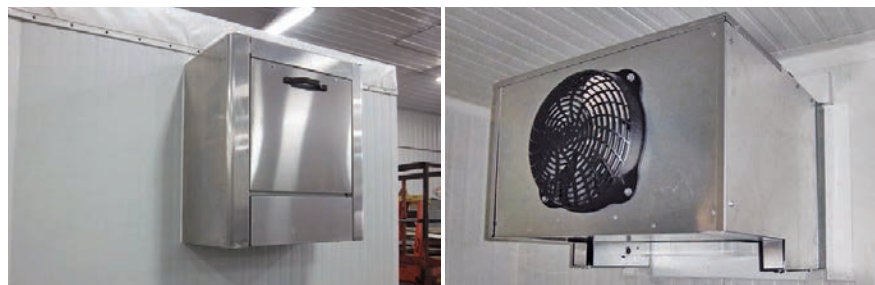
Figure 29. Side-mounted, self-contained refrigeration unit (evaporator and blower) shown from the outside (left) and inside (right) of the cooler. (Barr, Inc.)
