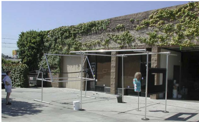
Visual 43: Construction at of new Esmeralda rig at Composite Components Company
