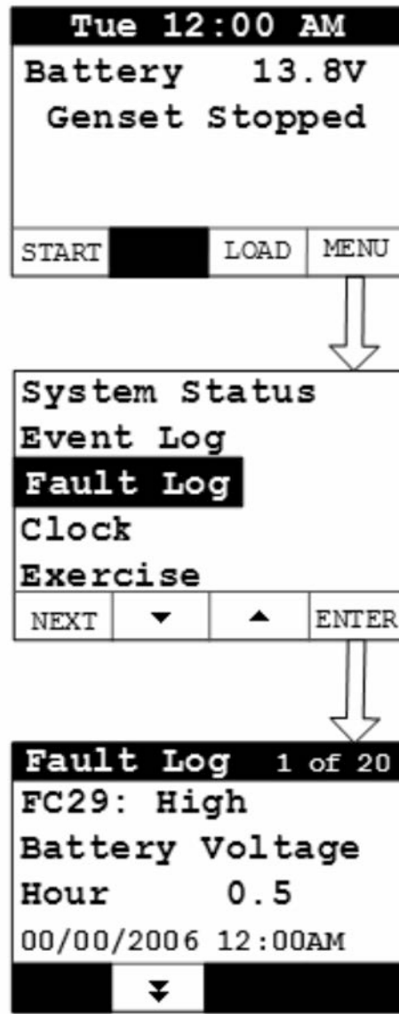
FIGURE 27. FAULT LOG SCREEN
