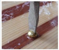
Install the vent screw in the insert nut and screw it into the hole until the top of the insert nut is flush with the deck. Unscrew the vent screw and allow the epoxy to fully cure. Sand any excess epoxy even with the top of the deck.
