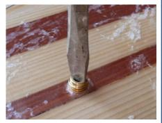
Drill a 13/32" hole in the deck and screw the nut flush with the deck. Remove the nut and turn it over.
