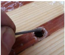
Coat the top of the drilled hole to make sure there is a good seal between the glass and wood.
