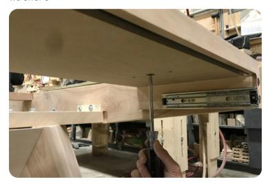
Repeat operations 15 and 16 for the second short apron or, for a product with a drawer, fix the drawer's box to the crossmember using 1/4"-20 x 1/2" machine screws and machine screws 1/4"-20 x 1/2" (round head). to the apron.
