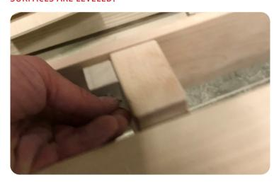
Fix this same short apron to the long base frames with 1/4"-20 x 1 1/2" machines screws and 5/16" flat wa sher s
