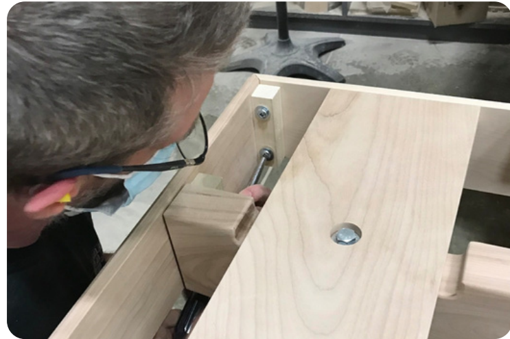
10 Fix the first short apron's corners to the long aprons with 1/4"-20 x 1 1/2" machines screws and 5/16" flat washers
