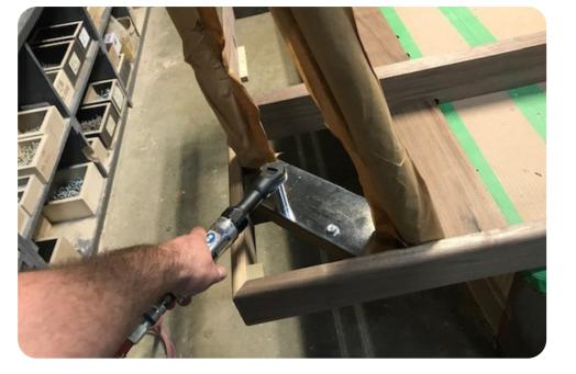
**13** Install the legs with 3 8"-16 x 1" hexagonal bolts and 7/16".flat wachers.. WITH HELP, TURN OVER THE ASSEMBLED TABLE AND PUT IT IN PLACE.
