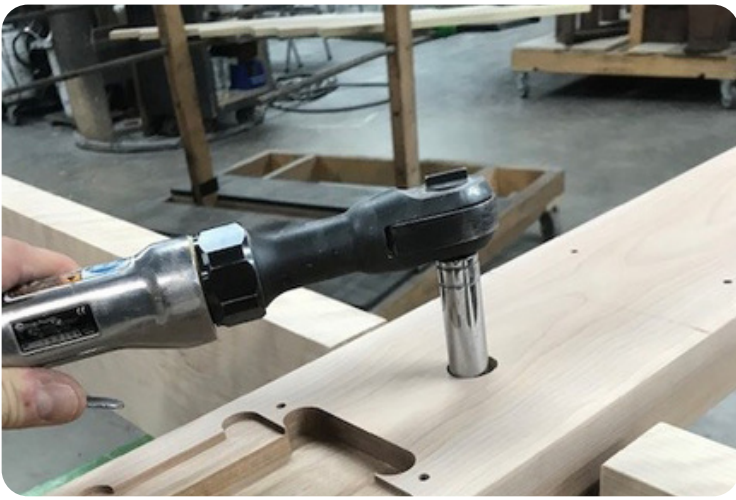
7 Fix the net crossmember with 3/8"-16 x 1 3/4" hexagonal bolts and 13/32" flat washers.
