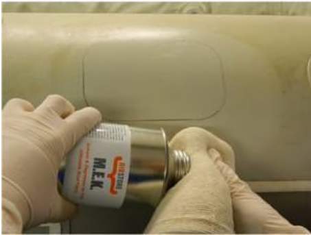
Clean and prime the repair area prior to applying the adhesive
