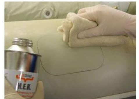
Cleaning all excess glue from the repaired area
