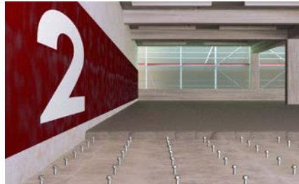
Parking garage reinforcement
