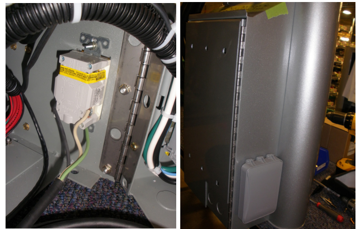
Figure 12. GFCI Receptacle Location - Reference Only
