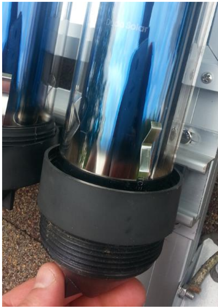
Screw bottom piece into tube holder to fasten tube tightly to manifold
