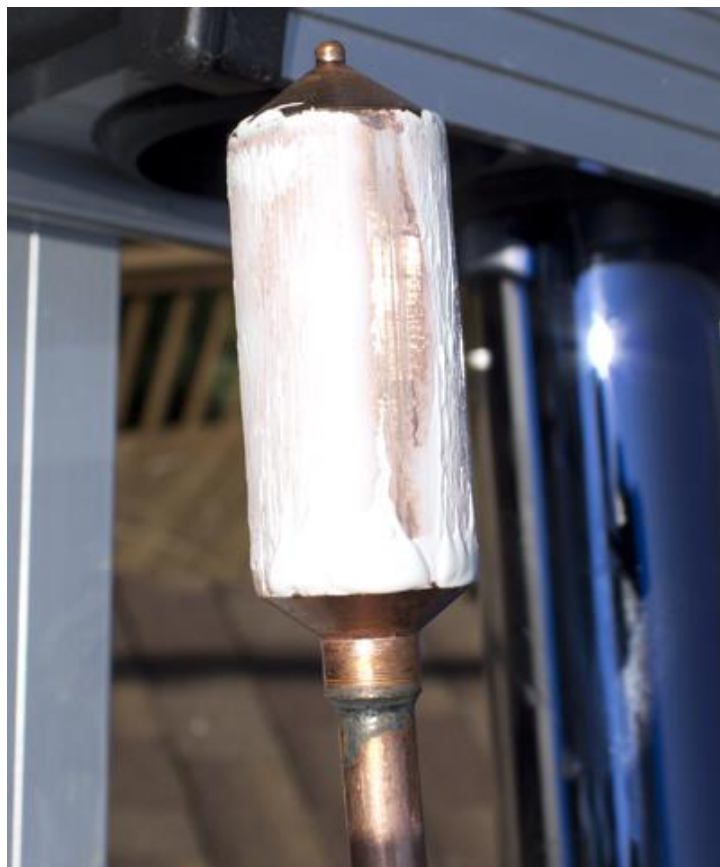
What Condenser Looks like After Removing from Manifold with Applied Thermal Paste
