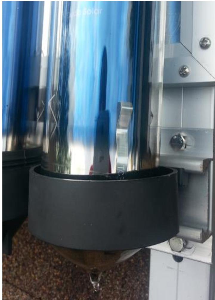
Snap top piece of tube holder into the bottom rail of the frame
