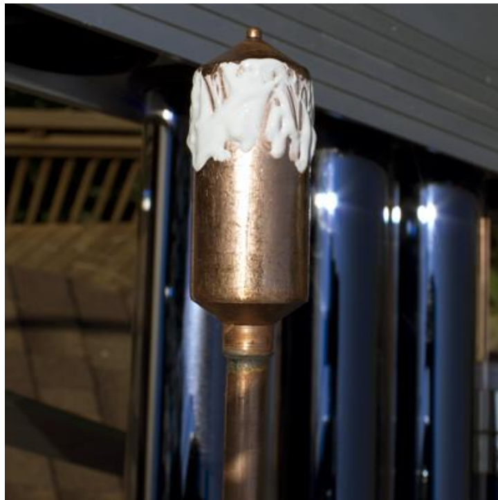
Coat the Condenser with Thermal Paste Prior to Insertion into the Manifold
