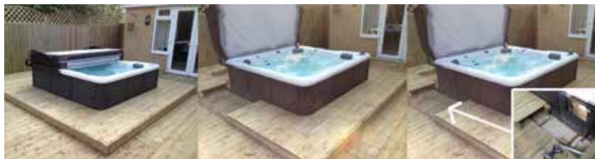
Ensure part of your decking can be removed in order to gain access for future repair or servicing
