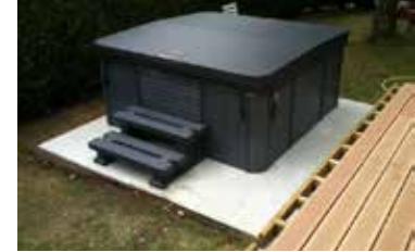
A 10-15 cm concrete base is ideal preparation for a hot tub.
