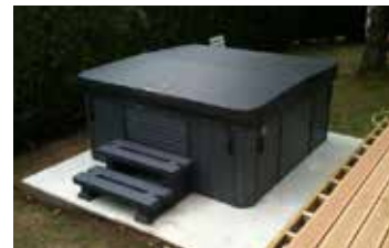
A 10-15 cm concrete base preparation for a acrylic Plug & Play hot tub.
