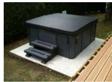
A 10-15 cm concrete base is ideal preparation for a hot tub.
