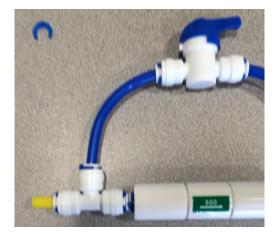
4. After assembling the flush valve, connect back to the TI filter waste water line.
