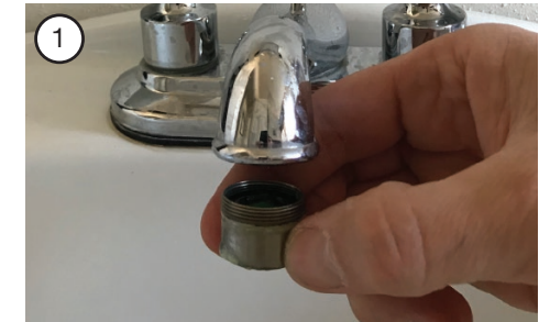
Remove the existing aerator on the sink faucet.
