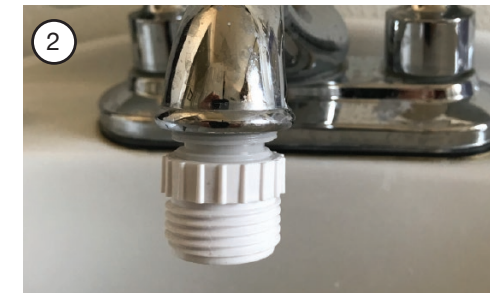
Thread-in the two-piece sink faucet adapter.
