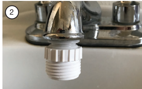
2 Thread-in the two-piece sink faucet adapter.
