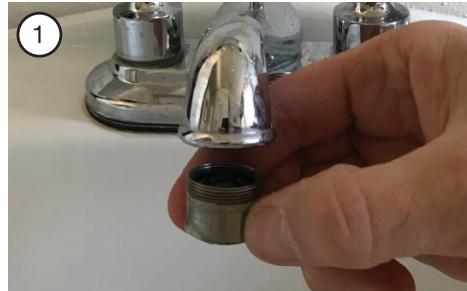
1 Remove the existing aerator on the sink faucet.
