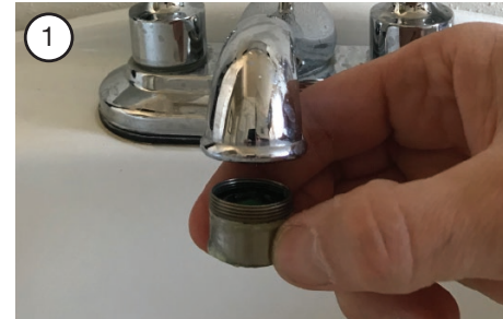
Remove the existing aerator on the sink faucet.
