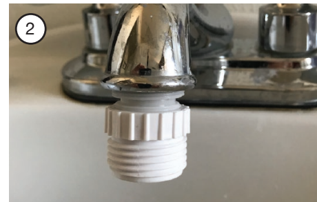
Thread-in the two-piece sink faucet adapter.
