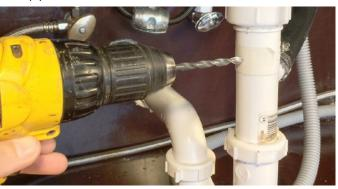
Step 5 – Align the Drain Saddle with the new hole in the drain pipe using a screwdriver through the Drain Saddle. Attach the solid Semicircle Bracket to the Bracket with the  $\frac{1}{4}$ " hole and loosely tighten the nuts by hand.
