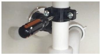
**Step 6** – Tighten the 2 screws and nuts using a Phillips screwdriver and 7/16" open-end wrench.
