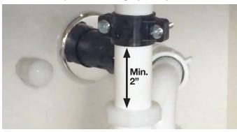
**Step 4** – Use a ¼" drill bit to make a hole in the drain pipe where you marked it on the masking tape. Remove the masking tape and clear any plastic burs/shavings from around the new hole in the drain pipe.
