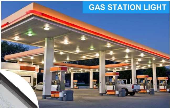
GAS STATION LIGHT
