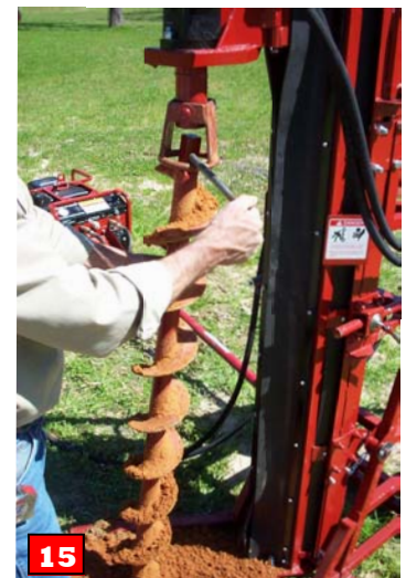
15 Continue procedure until lead auger is removed.
