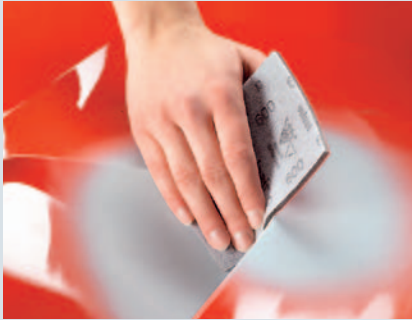
Final sanding of filler at hard to get at areas
