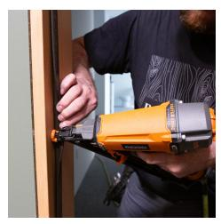
**Step 8.** Fasten the jamb to the stud on the hinge side and then the strike side, with nail gun or screws (screws recommended). If using screws, use the holes you pre-drilled in step 2.
