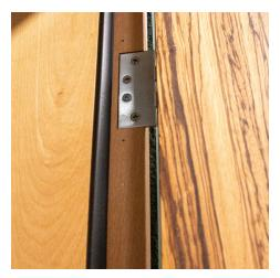
Step 5. Pre-drill holes for jamb screws if using screws. Jamb screws should go behind the weatherstripping or behind the hinges to better conceal them. If you have a very large door, an additional jamb screw should be placed on the jamb, parallel to the hinges. (If using nails, no pre-drilling is necessary).
