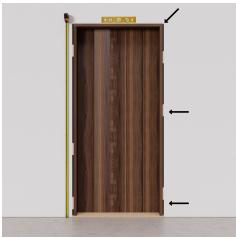
**Step 6.** Use mallet to ensure the unit is plumb. Check with a level and measuring tape to ensure that the unit is square and plumb.
