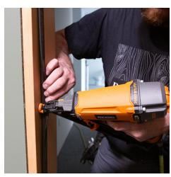
**Step 8.** Fasten the jamb to the stud on the hinge side and then the strike side, with nail gun or screws (screws recommended). If using screws, use the holes you pre-drilled in step 2.
