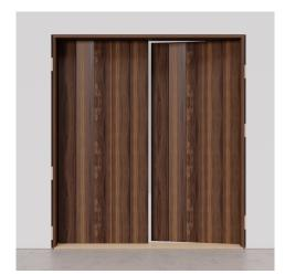
**Step 9.** Ensure the doors fit correctly by closing them and adjusting shims for the best fit and even gaps. Maintain an equal gap between door slabs at top and bottom. Adjust using shims/hinges until gapping is uniform, then secure hinges. Finally, check for any binding issues.
