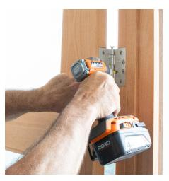
**Step 8.** Use the airbags to line up the hinges on the door and jamb, then set the pin in place. You may need to continue adding shims at this point. Once all hinges are in place, tighten the screws.
