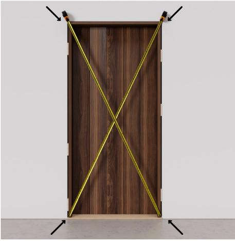
**Step 6.** Use mallet to ensure the unit is plumb. Check with a level and measuring tape to ensure that the unit is square and plumb.
