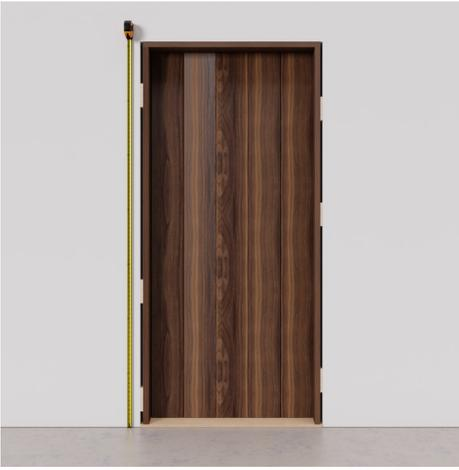
**Step 12.** Check both sides of the jamb for plumb again with a level.
