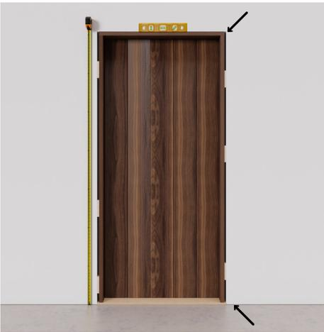
**Step 10.** Check both sides of the jamb for plumb again with a level.
