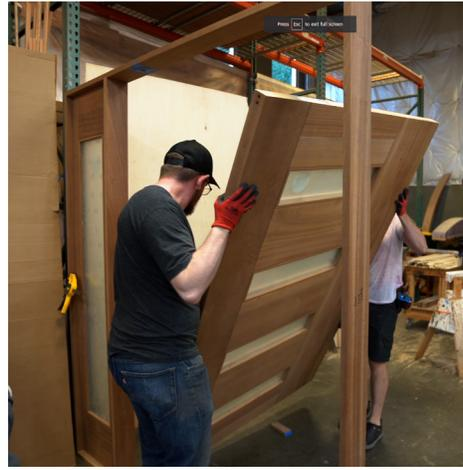
**Step 8.** The door can easily be placed by first lifting the oval spindle on the M+ bottom pivot into the notch in the floor plate. It is important that the door is set in its open position, so the oval spindle should be rotated into that direction. The Allen wrench is a useful accessory to accomplish this. Do not set the door on the pivot in the closed position. It will not work.
