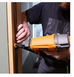
**Step 11.** Fasten the jamb to the stud on the hinge side and then the strike side, with nail gun or screws (screws recommended). If using screws, use the holes you pre-drilled in step 2.
