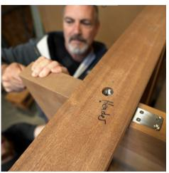
**Step 9.** After the door is placed on the bottom pivot, extend the top pivot by turning the Allen wrench (included with your FritsJurgens packaging). Turn the Allen wrench in the hole at the top of the door (approximately eight times).
