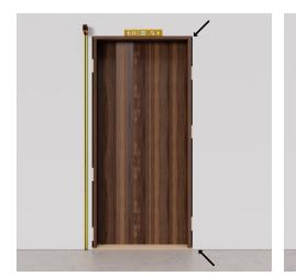
**Step 10.** Check both sides of the jamb for plumb again with a level.
