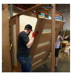
**Step 8.** The door can easily be placed by first lifting the oval spindle on the M+ bottom pivot into the notch in the floor plate. It is important that the door is set in its open position, so the oval spindle should be rotated into that direction. The Allen wrench is a useful accessory to accomplish this. Do not set the door on the pivot in the closed position. It will not work.
