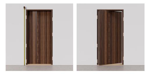
**Step 12.** Check both sides of the jamb for plumb again with a level.
