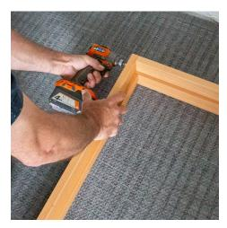
**Step 1**. Assemble the jamb using the pre-drilled holes.
