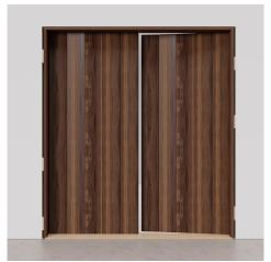
**Step 9.** Ensure the doors fit correctly by closing them and adjusting shims for the best fit and even gaps. Maintain equal gap between door slabs at top and bottom. Adjust using shims/hinges until gapping is uniform, then secure hinges. Finally, check for any binding issues.
