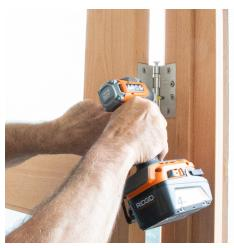
Step 8. Use airbags so that the doors are flush with hinge prep in the jamb. Line up the hinges on the door with the hinges on the jamb, one hinge pair at a time, then set the pin. You may need to continue adding shims at this point. Once all three hinges are pinned, you can add the rest of the hinge screws but do not fully tighten them until after step 9.
