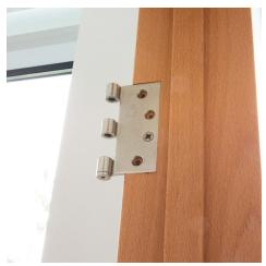
**Step 7.** Screw the hinges onto the jamb and onto the door slabs with one screw per hinge. Do not fully tighten the screw so that you can adjust the hinges if necessary.
