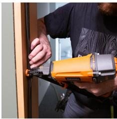
**Step 10.** Screw or nail the jamb to the studs behind the weatherstripping, so that the screws are concealed. Screws recommended.
