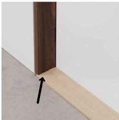
**Step 3.** Spread silicone between the threshold and jamb legs to prevent water damage.
