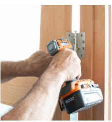
**Step 8.** Use airbags so that the doors are flush with hinge prep in the jamb. Line up the hinges on the door with the hinges on the jamb, one hinge pair at a time, then set the pin. You may need to continue adding shims at this point. Once all hinges are in place, tighten the screws. Insert all hinge screws.
