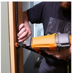
**Step 10.** Screw or nail the jamb to the studs behind the weatherstripping, so that the screws are concealed. Screws recommended. Place shims where you screw through the jamb.
