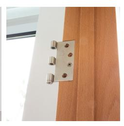
**Step 7.** Screw the hinges onto the jamb and onto the door slabs with two screws per hinge. Do not fully tighten the screw so that you can adjust the hinges if necessary.
