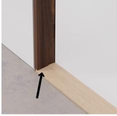
**Step 3.** Spread silicone between the threshold and jamb legs to prevent water exposure.
