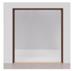
**Step 4.** Test fit the unit in the rough opening. If it fits, remove it from the opening and apply at least three heavy beads of silicone all the way across where the threshold will make contact with the sub-floor.
