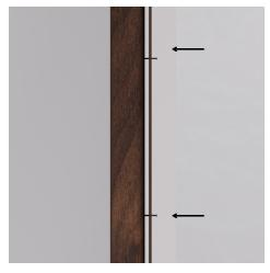
**Step 11.** Attach the astragal over the gap between the doors using screws, centering it for an optimal fit.
