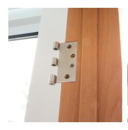
**Step 5.** Screw the hinges onto the jamb and onto the door slabs with two screws per hinge. Do not fully tighten the screw so that you can adjust the hinges if necessary.
