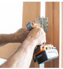
**Step 6.** Use the airbags to line up the hinges on the door and jamb, then set the pin in place. You may need to continue adding shims at this point. Once all hinges are in place, tighten the screws. Insert all hinge screws.
