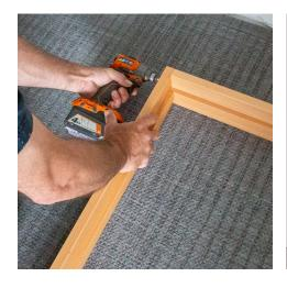
**Step 1**. First, measure and confirm the rough opening size. Next, assess the assembled jamb dimensions to ensure it fits the rough opening accurately.
