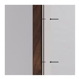
**Step 10.** Attach the astragal over the gap between the doors using screws, centering it for an optimal fit.
