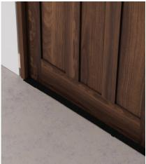
**Step 9.** Cut and test fit the aluminum threshold. Once the threshold has been test-fitted, apply at least three beads of silicone to the subfloor and set the threshold firmly in place.
