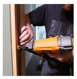
**Step 8.** Screw or nail the jamb to the studs behind the weatherstripping, so that the screws are concealed. Screws recommended. Place shims where you screw through the jamb.
