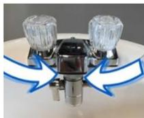
Finally, the diverter valve may simply not be tightened enough. Hold both the diverter valve and its collar and turn them together to tighten it further.
