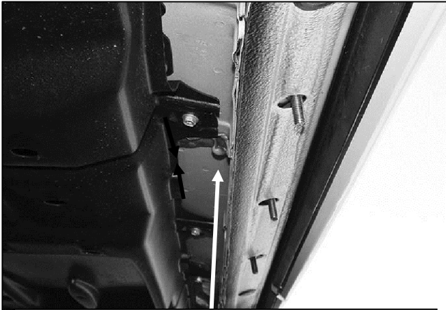
(Fig 3) Scrape excess body sealant as necessary from all locations before installing
