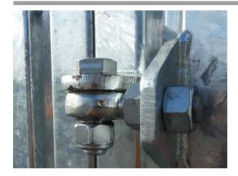
The gates swing on 20mm greasable spherical rod end bearings giving a smooth gate action and the ability to adjust your gates if they ever sag.
