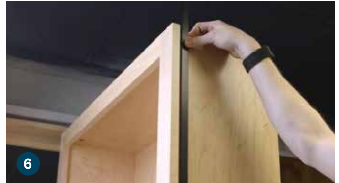
Position the top bracket one finger-width from the top of the door and secure with (2) 1/2" Phillips head screws.
