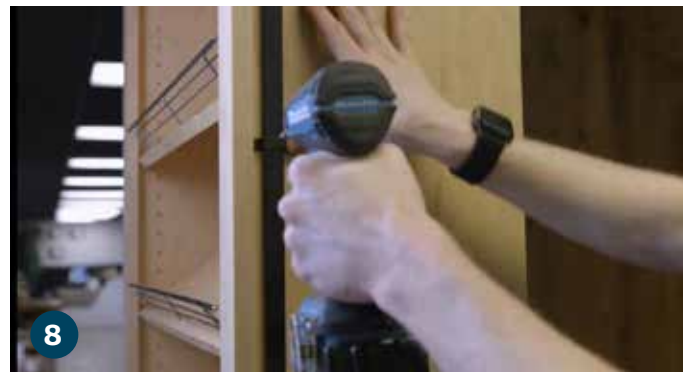
Position the center bracket halfway between the two brackets and secure with (2) 1/2" Phillips head screws.
