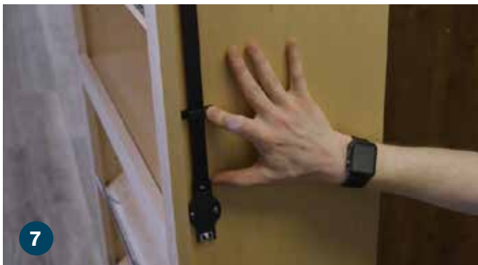
Secure the bottom bracket four fingers above the lock using (2) 1/2" Phillips head screws.
