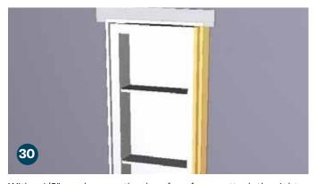
With a 1/2" overlay over the door face frame, attach the right side casing using a brad nailer and finishing nails.
