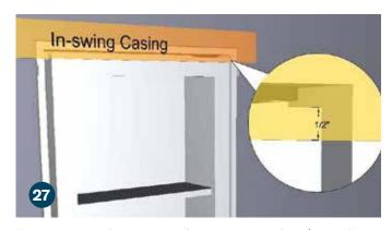
For an in-swing door, position the top casing with a 1/2" overhang on the face frame of your door and attach using a brad nailer and finishing nails.
