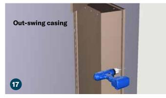
Using a 1/8" drill bit pre-drill and countersink five holes into the left support face frame. This will make it easier to attach the left side casing.
