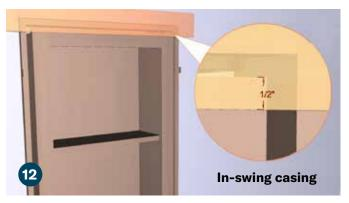
For an in-swing door, position the top casing with a 1/2" overhang on the face frame of your door. Attach using a brad nailer.
