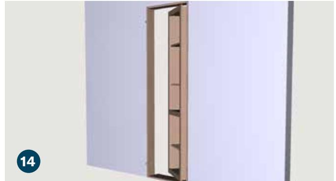
Test the in-swing to ensure the door opens and closes smoothly.
